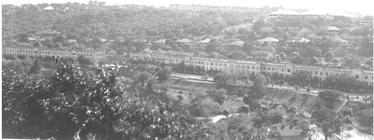
Bottomside Barracks and Officer Housing at Ft Mills, Corregidor, seen from Malinta Hill
